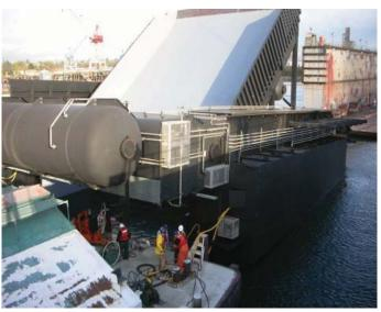
Removable Surface Weir (RSW) for Ice Harbor Dam. Photo: US Army Corps of Engineers.
